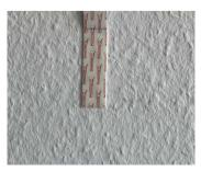
3. Press down evenly over the entire strip for at least 5 seconds, and only then remove the protective foil.
